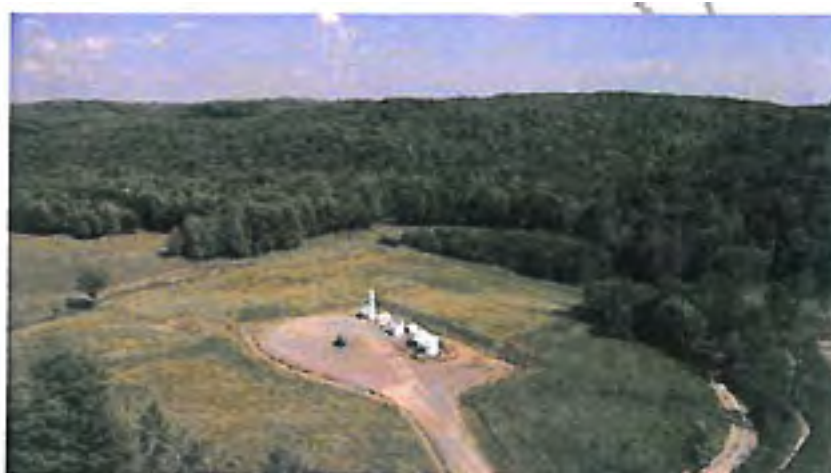
Multi-well pad (source: eCorp)
